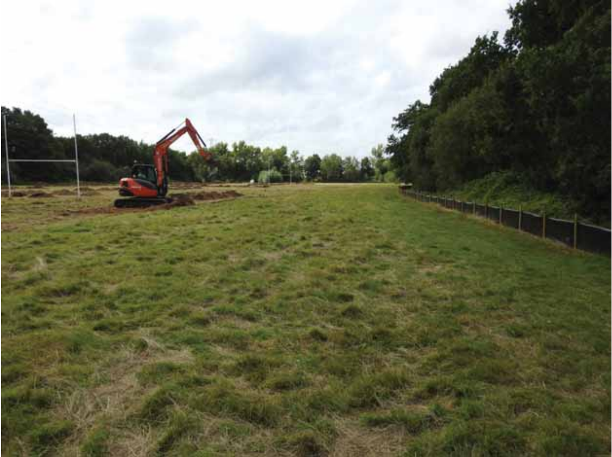
Plate 63: Viewing the site from north-east. Machine carries out back-filling of finished trenches.
